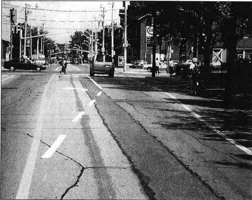
Figure 3. Left-turn lanes are provided at signalized intersections to reduce congestion and make left turns easier for cyclists.
