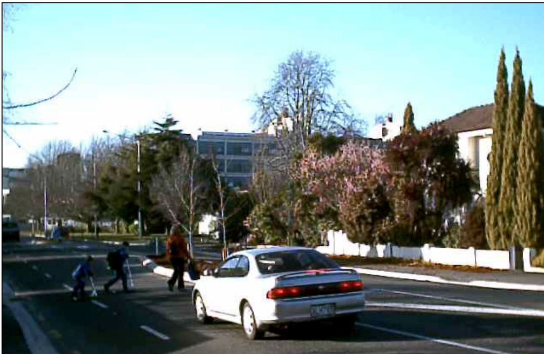
Figure 4: Crossing the road is easier for pedestrians and cyclists with the addition of islands. Trees on the islands will grow to help shorten the view and reduce speeds.
