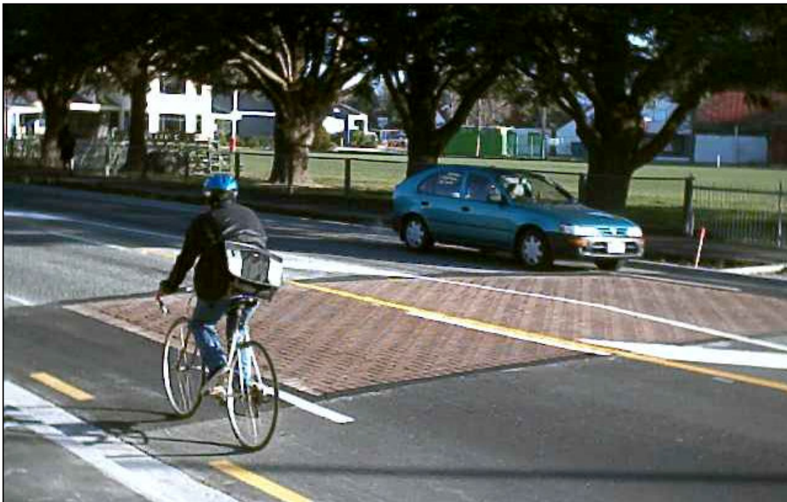
Photo 3: Threshold treatments at each end of Creyke Road signify to road users that this is no ordinary street. Medbury School in the background.
