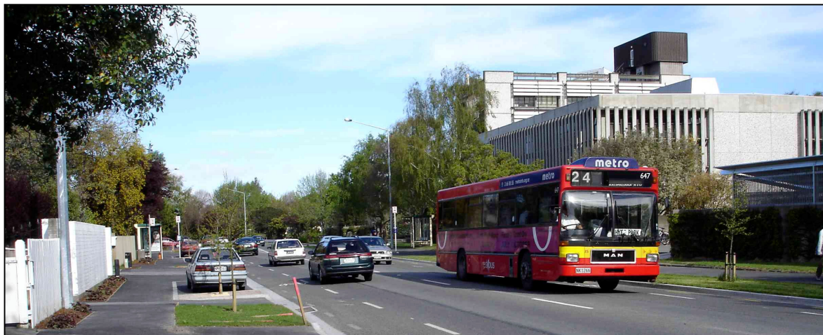
Figure 5: Creyke Road before (top) and after (bottom) reconstruction
