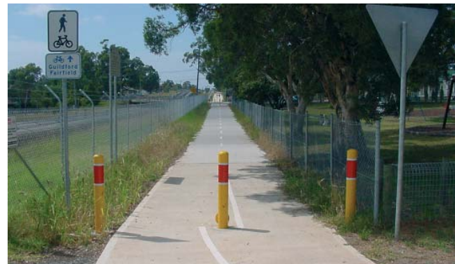
Figure 8 - Example of preferred bollard treatment to prevent motor vehicle access (courtesy RTA, NSW)
