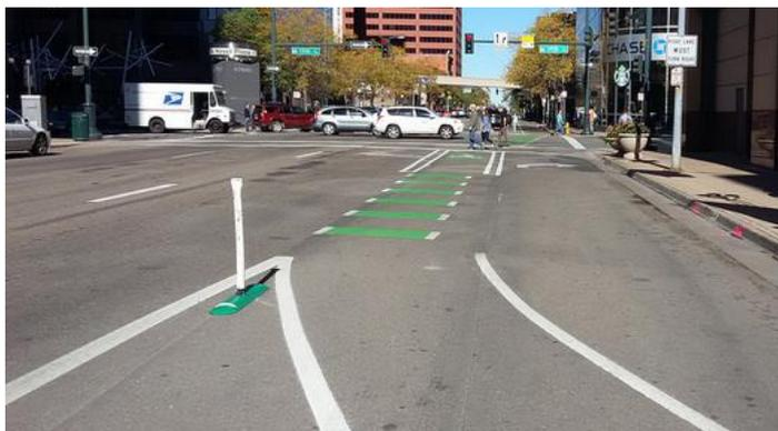
Figure 4: Separated cycleway transitions to cycle lane between through and right turn lanes, Lawrence St, Denver
