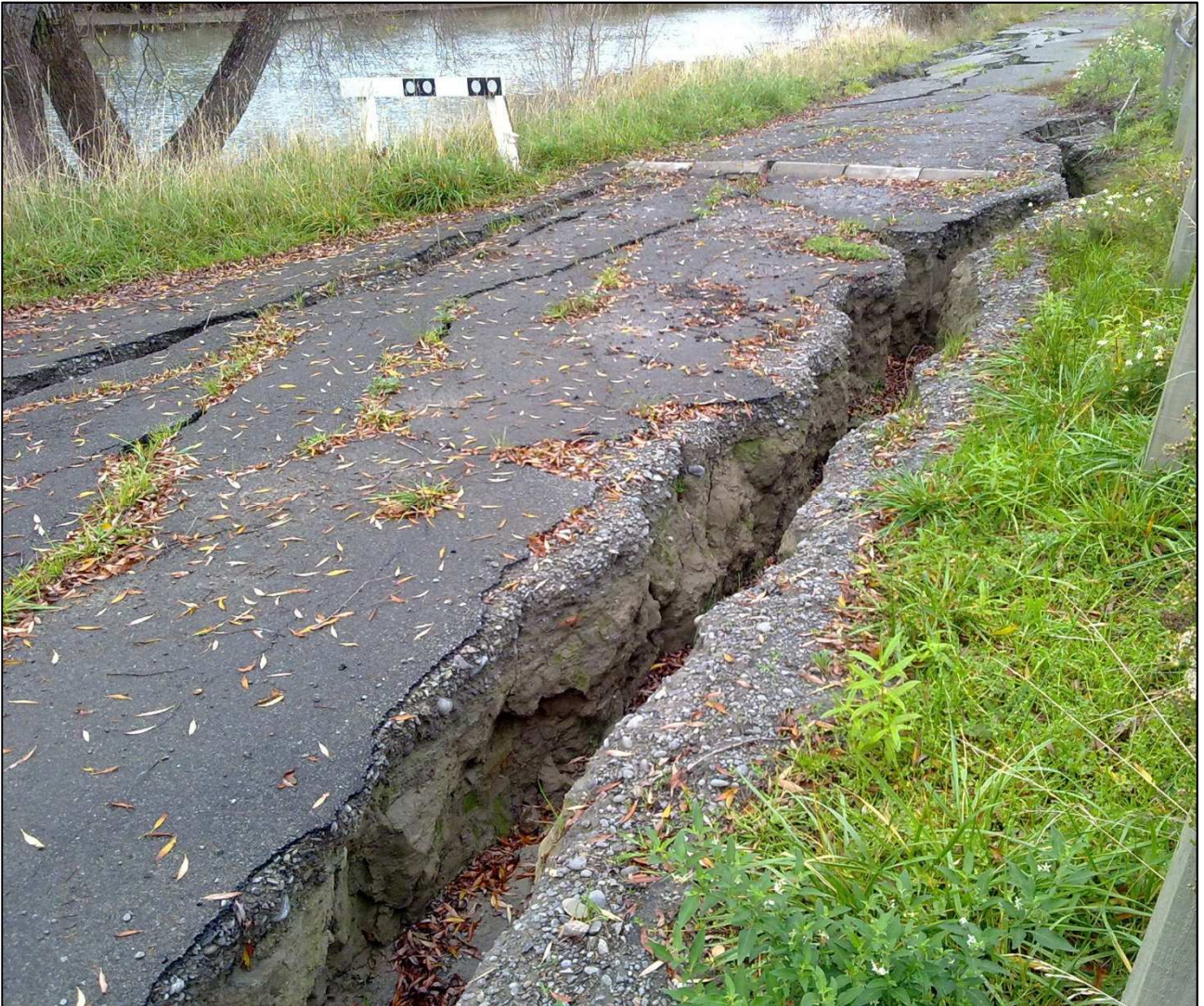
Figure 1: Example of road damage following 2010-11 Canterbury quakes
