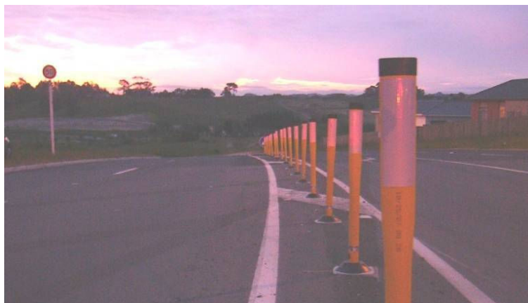
Figure 5: Flexible bollards (Silverdale)
