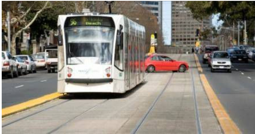
Figure 4: Raised separators (Melbourne)
