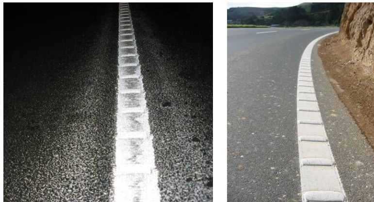
Figure 3 : Textured road marking in Dunedin; 4 mm urban (left) and 7 mm rural (right)
