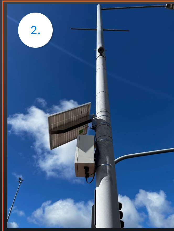
Portable machine Duration: 24 hr – 2+ mo
