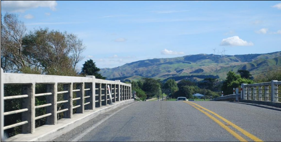
Figure 62: Many railway overbridges have inadequate shoulder width and may require clip-on bridges on each side for cycling safety (photo: Jonathan Kennett)
