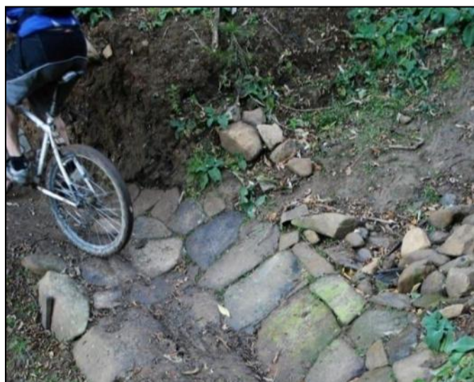
Figure 28: Rock armoured path - Nichols Creek Track, Dunedin (photo: Kennett Brothers)
