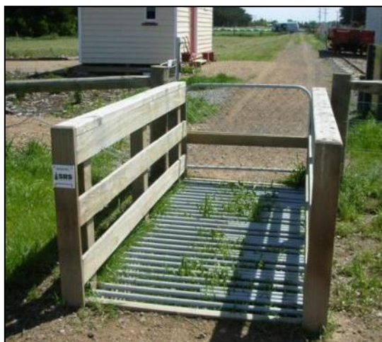
Figure 70: Gate added – a poor solution for cycling
