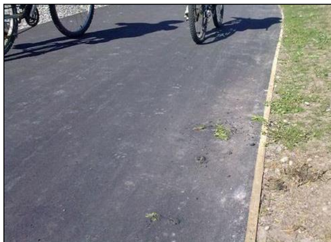
Figure 106: Vegetation growing through new asphaltic concrete path; good construction specifications and contract supervision are required
