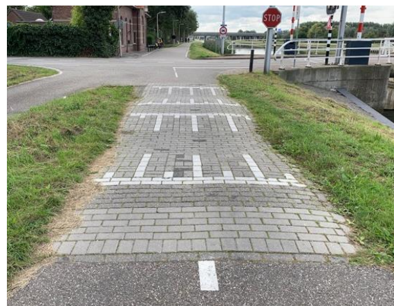
Figure 7-2: Paver concave multi-speed bump, Arkel The Netherlands (image: J. Lieswyn)
