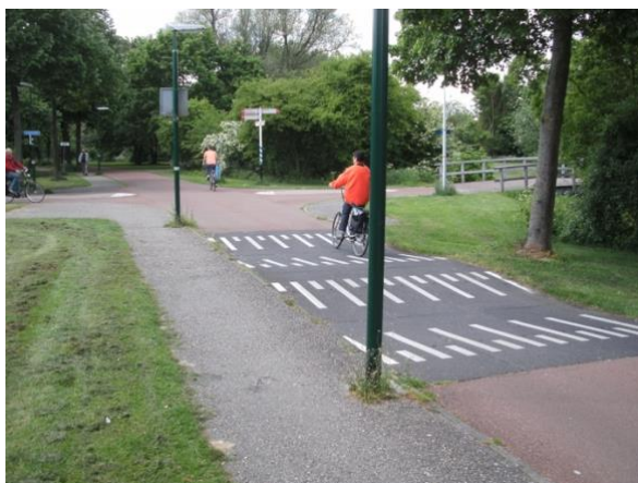
Figure 7-1: Asphalt concave multi-speed bump, Houten The Netherlands (image: G. Koorey)
