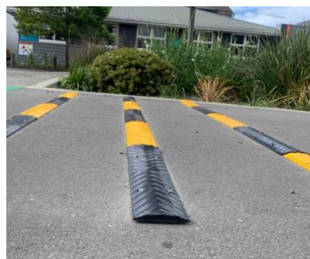
Figure 5-1: Rumble strip detail
