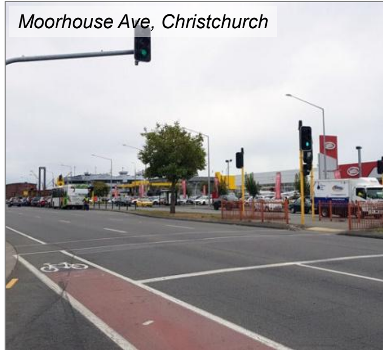
Two-stage pedestrian crossings
