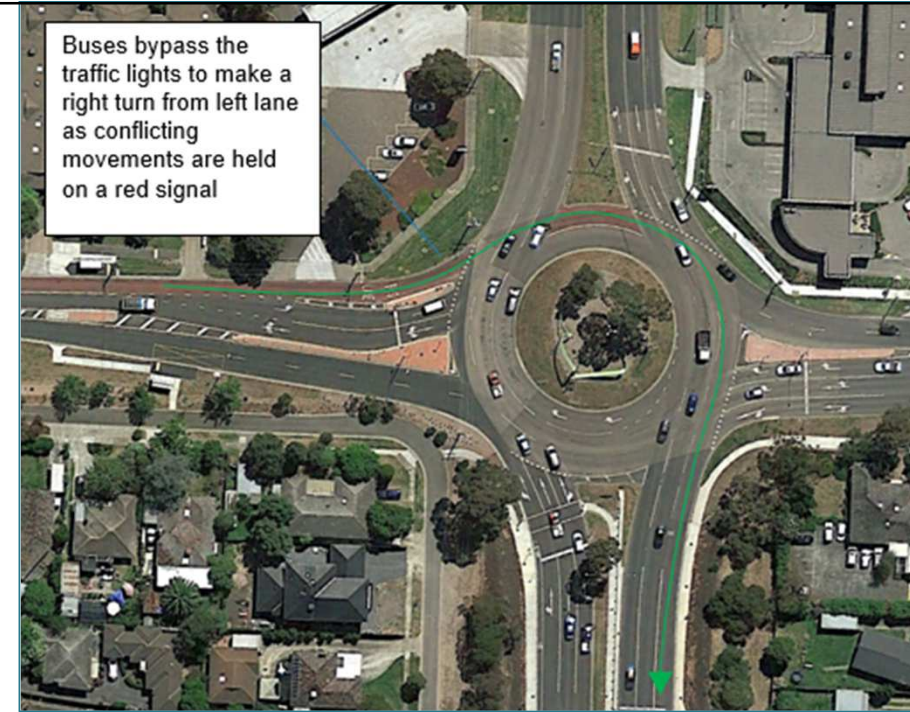
Williamsons/Porter roundabout, Melbourne
