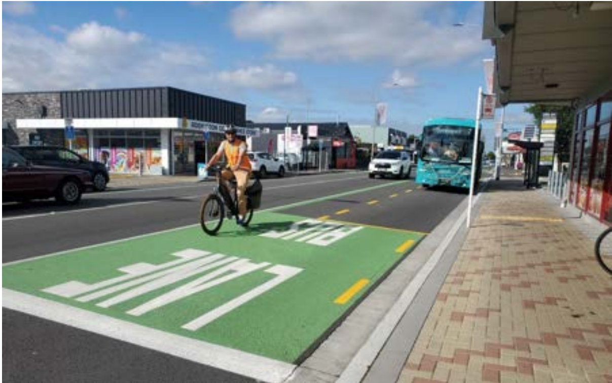
Figure 25-1: Bus-cycle lane, Lincoln Rd, Christchurch
