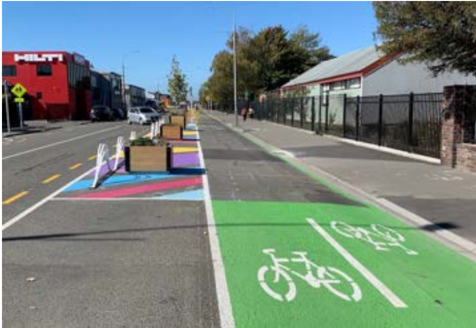
Figure 19-1: 2-way separated cycleway, Ferry Road, Christchurch
