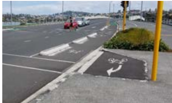
Figure 32-3: Jug handle at signalised crossing, Auckland
