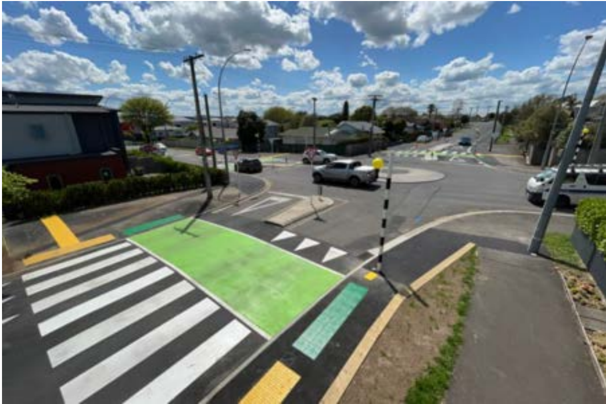
Figure 30-1: Dual crossing on raised safety platform at roundabout, Queens Ave / Killarney Rd, Hamilton
