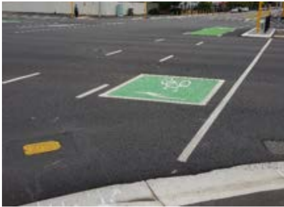
Figure 32-2: Hook turn box at signalised intersection, Christchurch
