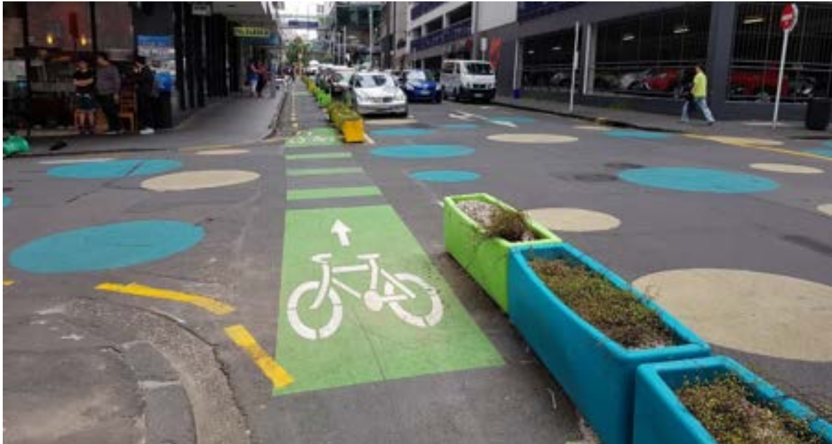
Figure 19-2: Contra-flow cycleway crossing side street, Federal Street, Auckland
