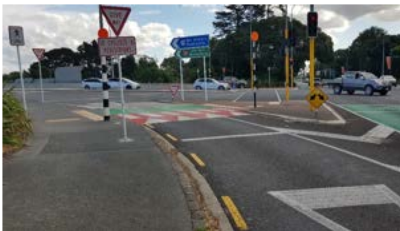
Figure 32-10: Dual pedestrian / cycle priority slip lane crossing, St Lukes Road, Auckland
