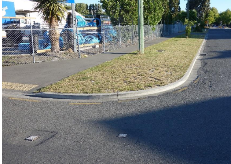
Figure 2: Superfluous no-stopping lines, as stopping within 6 m of an intersection is not allowed
