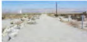
Top of 12' 0" wide independent fence with modular slope protection (left) and gentle road slope (right), view looking from Indian Canyon Drive.
