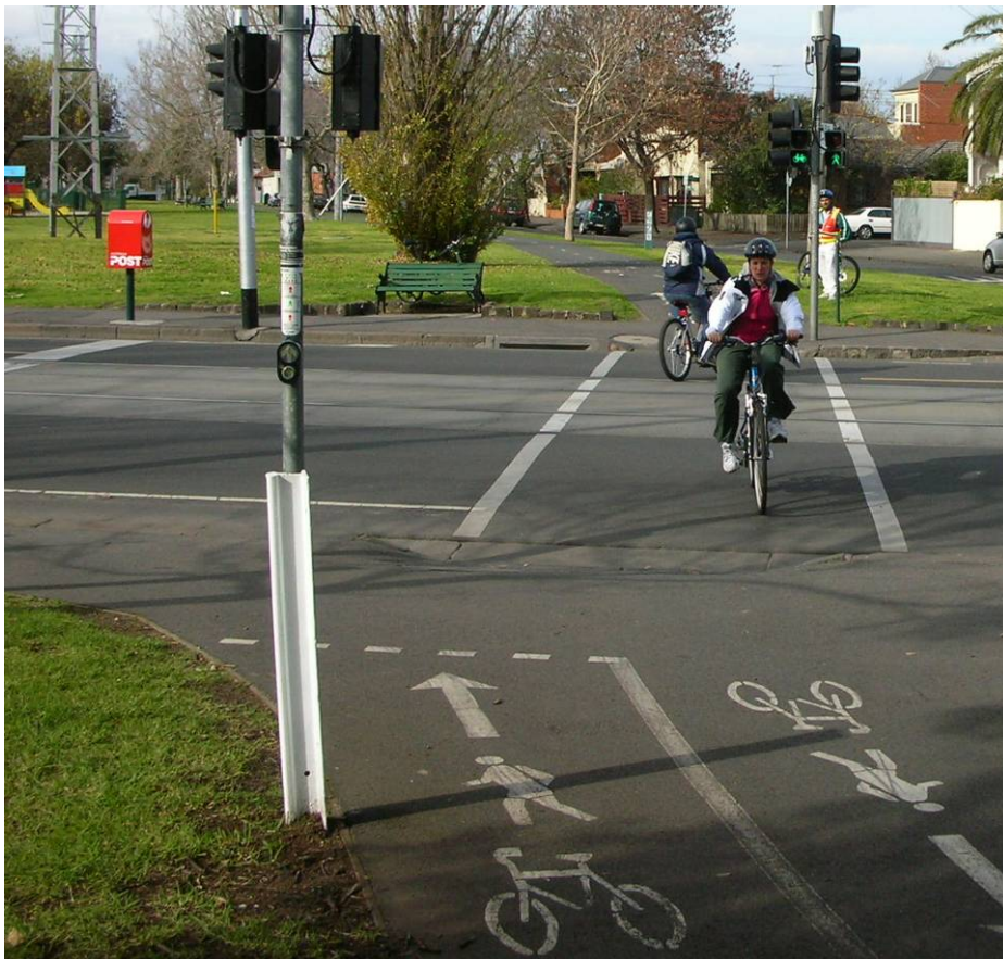
Figure 10: Signalised mid-block cycle crossing, Melbourne
