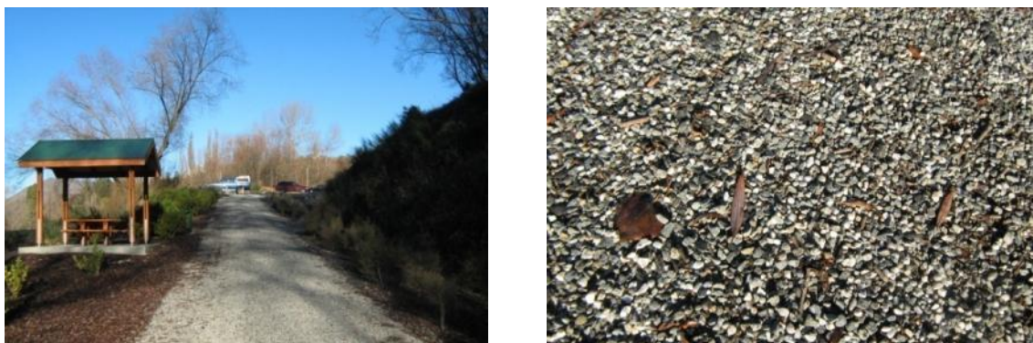
Figure 23 Chip seal path Queenstown
