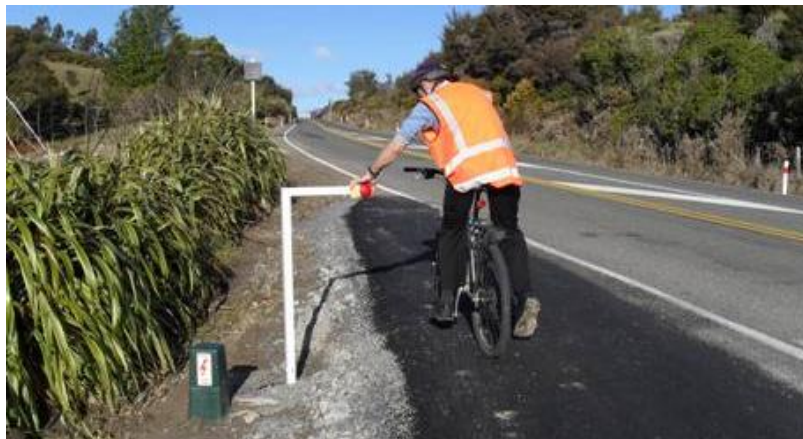
Figure 34: Push button activated warning sign at vertical crest, SH 60 near Nelson (photo: NZTA)
