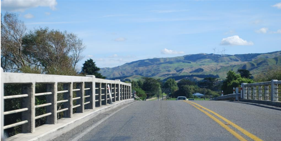
Figure 45: Many railway overbridges have inadequate shoulder width and may require clip-on bridges on each side for cyclist safety (photo: Jonathan Kennett)
