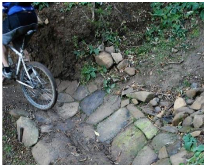
Figure 22: Rock armoured path - Nichols Creek Track, Dunedin (photo: Kennett Brothers)
