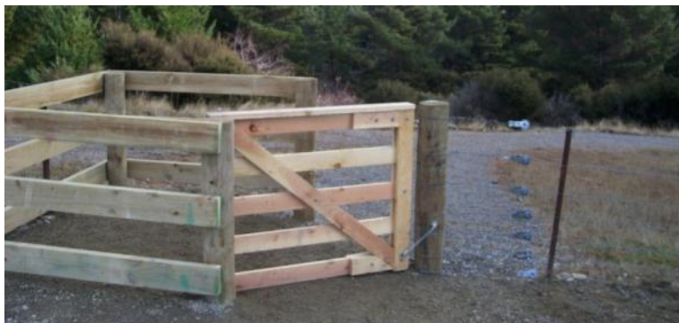
Figure 57: Kissing gate: Hawea Track; can be difficult for tandems and bikes with trailers
