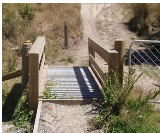
Figure 54: Cattle stop with good alignment, Port Hills (photo: Nick Singleton)
