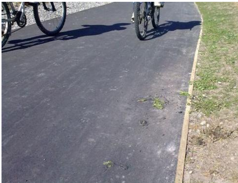
Figure 79: Vegetation growing through new asphaltic concrete path; good construction specifications and contract supervision are required
