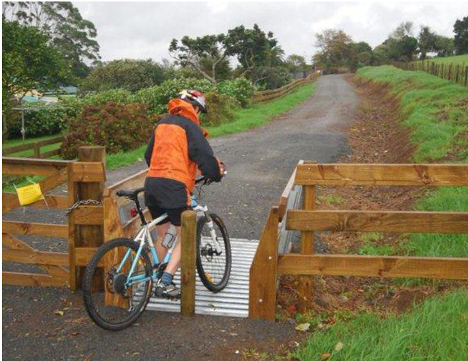
Figure 56: A central post and wing barriers help prevent motor-cycle access and reduce the likelihood of stock jumping the cattle stop (photo Jonathan Kennett)
