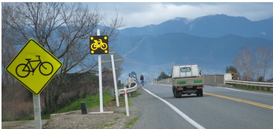
Figure 35: Inductive loop activated warning sign on narrow Appleby bridge, SH 60, near Nelson (photo: NZTA)
