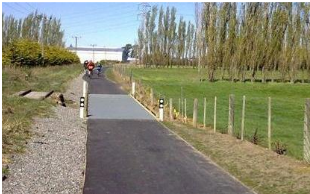
Figure 24: Asphaltic concrete section (and bridge) on the Little River Rail Trail at Hornby
