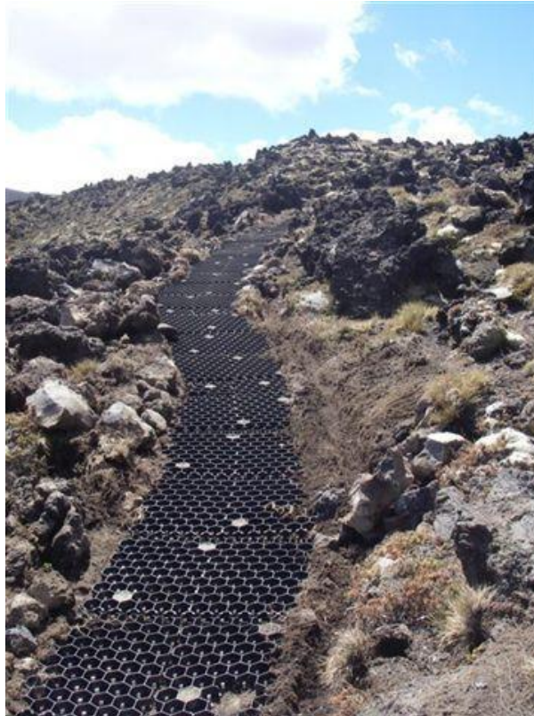
Figure 21: "Geomat" surface stabilisers, Tongariro National Park (photo: John Bradley)
