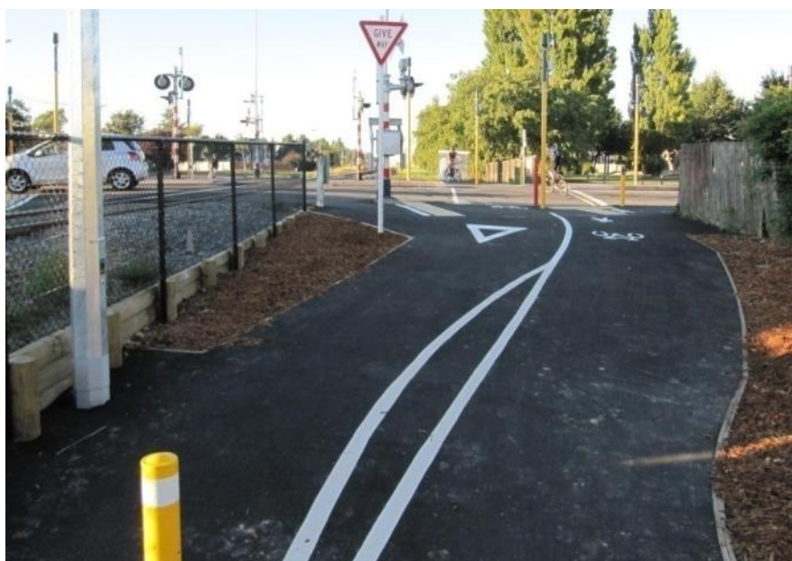
Figure 26: Bollards and painted markings as route end treatments, Railway Cycleway, Christchurch
