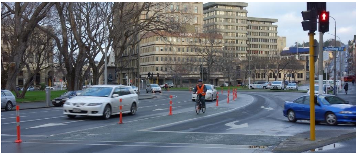
Figure 2: Short term measure utilising flexible bollards
