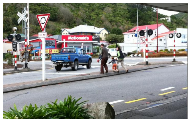
Figure 19: A family crosses the raised median "splitter" island at the Tainui Street roundabout
