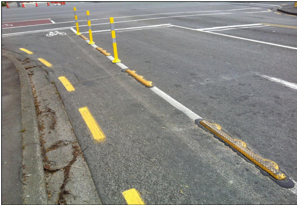
Figure 2: Strickland Street Riley separators and posts approaching intersection
