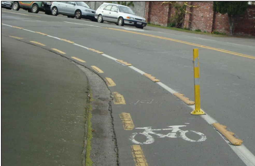
Figure 1: Riley separators and a vertical post installed on Kotare Street cycle lane line
