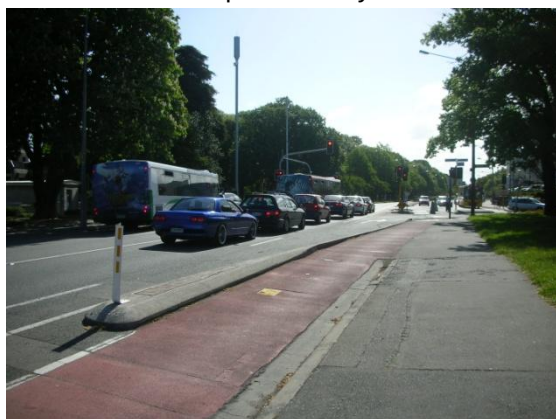
Contra flow kerb protected cycle lane, Christchurch
