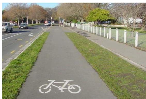
Two-way cycle path with kerb to carriageway (no parking) and berm to footpath, Christchurch
