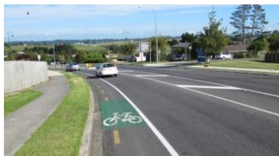
Kerbside cycle lane with colour highlight, white cycle logo and broken yellow no stopping lines, Auckland
