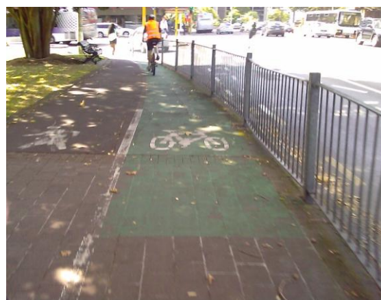
One-way cycle path with kerb to carriageway and paint line to footpath, Symonds St, Auckland
