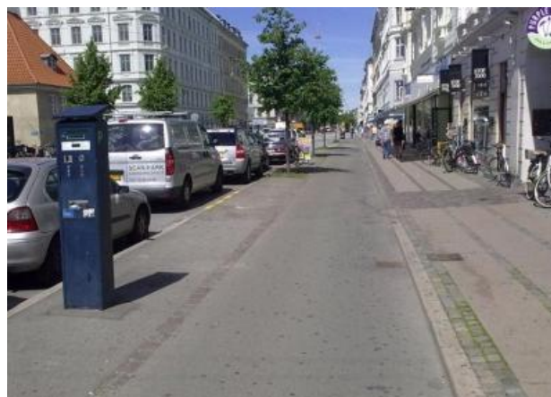
Danish cycle track with kerb zone for trees and parking meters, kerb and paver kerbing to footpath, Copenhagen
