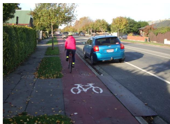
One-way cycle path with kerb to carriageway (with parking) and berm to footpath, Christchurch
