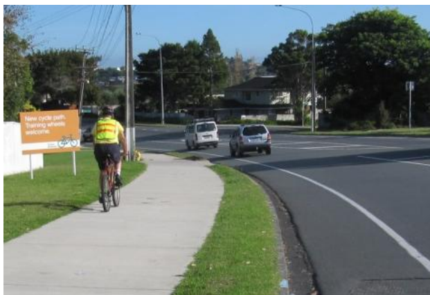
Shared path along road with cycle lane, North Shore
