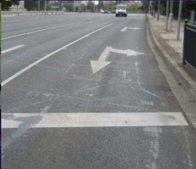
Inductive loop in road
