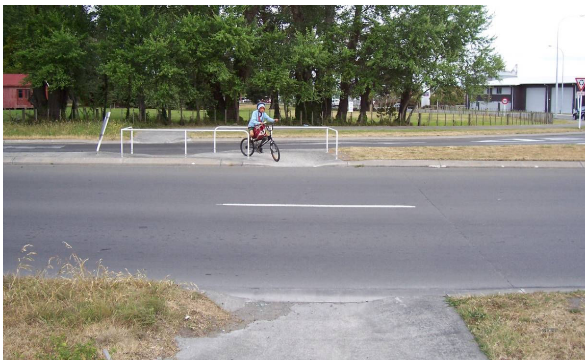
Figure 1: Crossing facility for the 100 km/h road . Roundabout located 30 m to the right.
