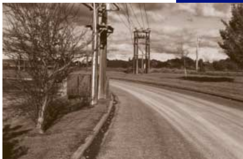
These power poles close by the roadside are a potential hazard for a vehicle leaving the road.
