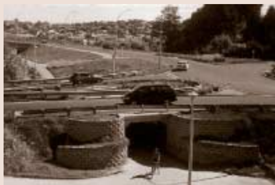
Underpass at multi-lane roundabout provides safety for cyclists and pedestrians
