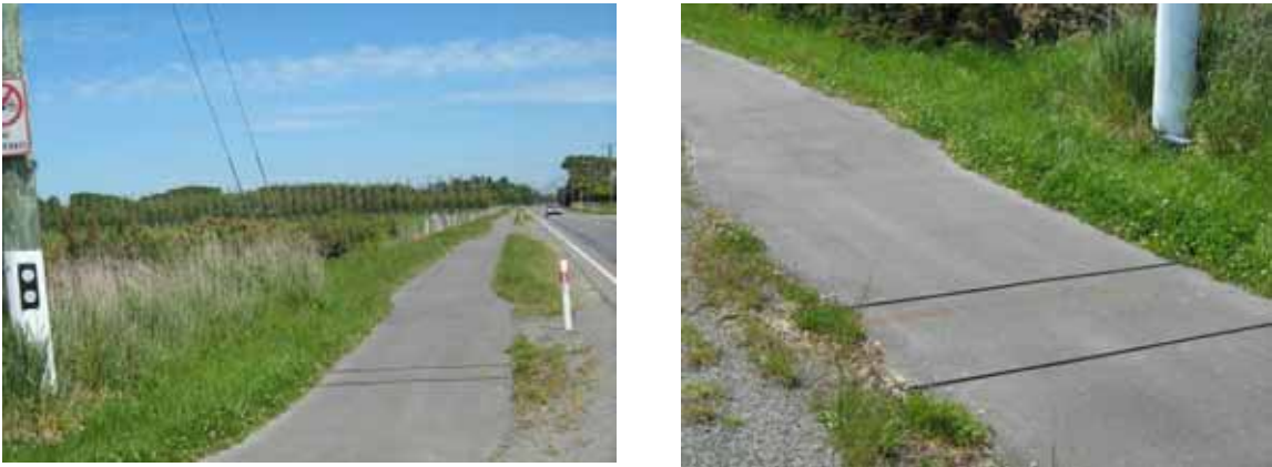
Figure A1 Typical off-road path counting installation
