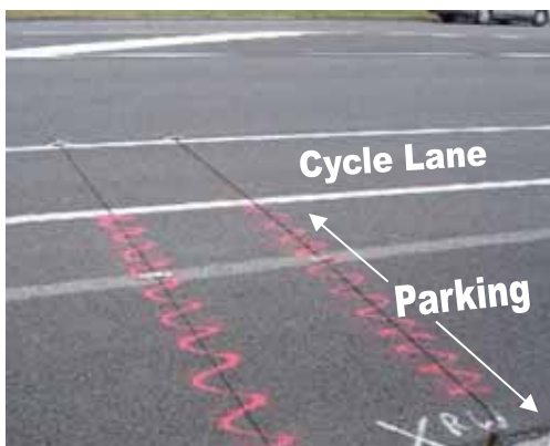
Figure A2 Spray painting tubes to discourage parking where parking demand is low
