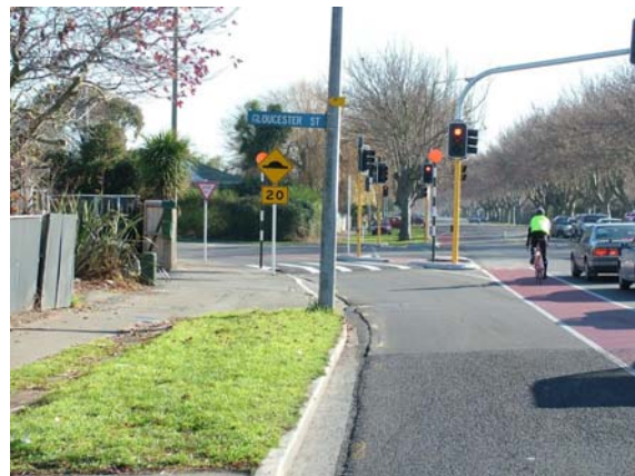
Figure 5: Pedestrian crossing on raised platform in slip lane
