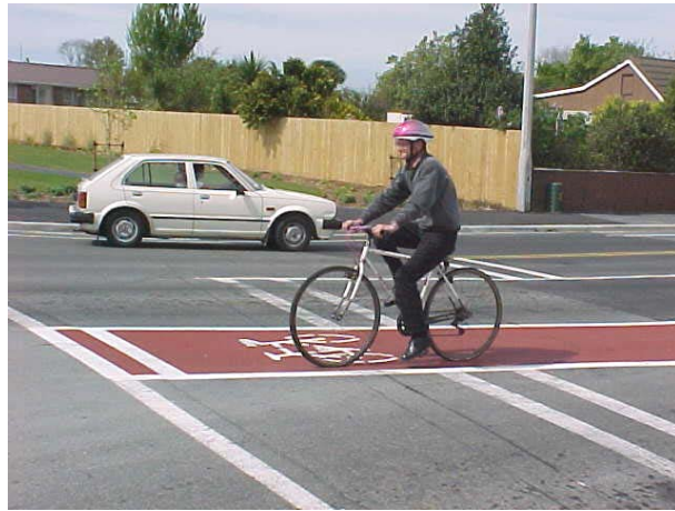
Figure 1: Advanced Stop Line
