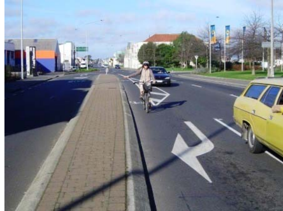
Figure 9: Gap for cyclists in chevron markings
